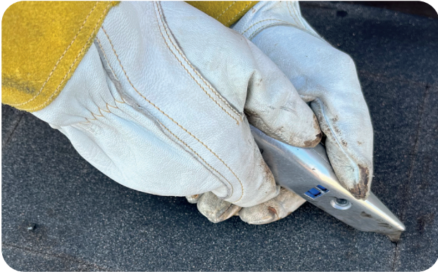
Remsa 25 x 500 mm skärs i underlaget.
